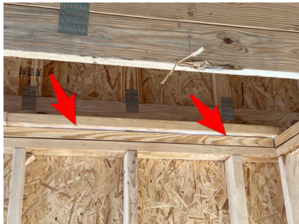
20: The exterior walls at the top plate need to be sealed in areas.
