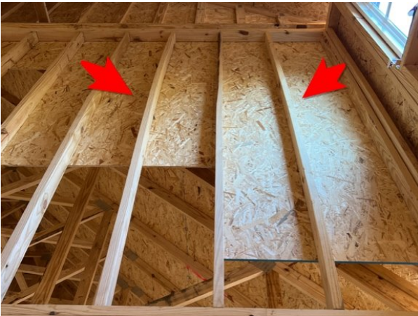
13: The upper interior wall adjacent to the attic had bowed studs.
