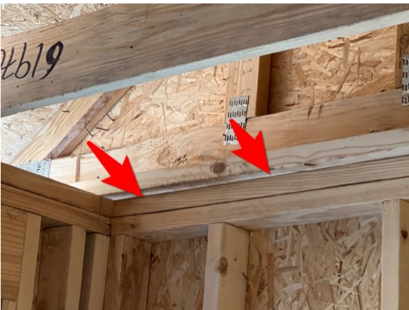
20: The exterior walls at the top plate need to be sealed in areas.
