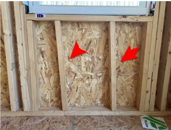
17: Leaning cripple studs under a window in an upstairs bedroom.
