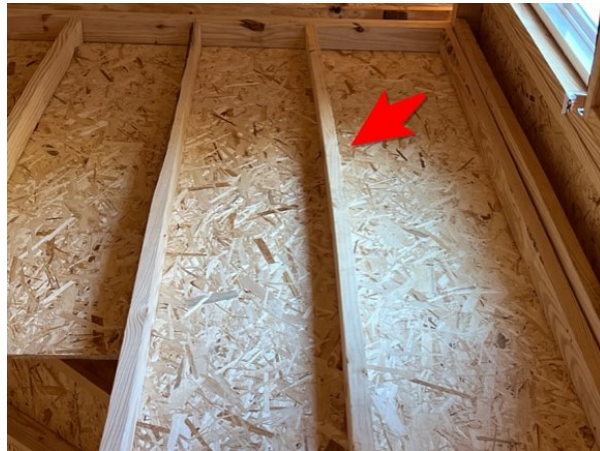
13: The upper interior wall adjacent to the attic had bowed studs.
