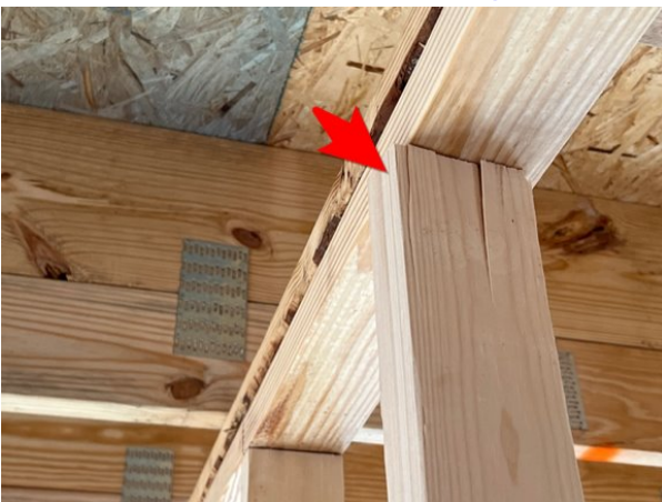
21: Twisted/loose stud in the upstairs back right bedroom.
