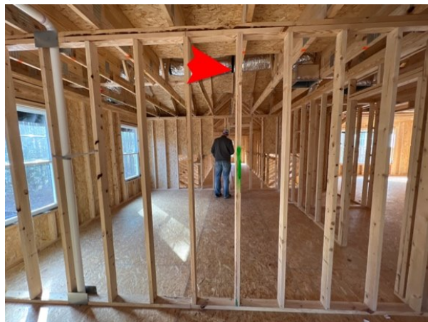
21: Twisted/loose stud in the upstairs back right bedroom.
