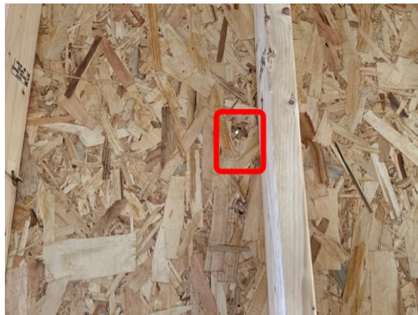
16: Missed nails noted in several areas on the exterior walls that need to be sealed.
