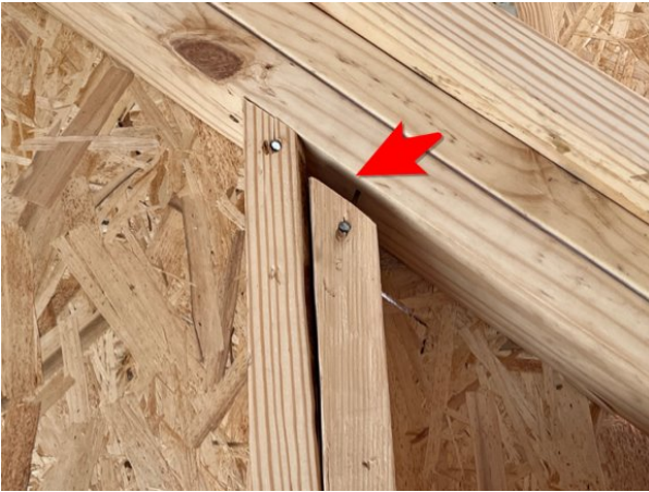
20: The exterior walls at the top plate need to be sealed in areas.
