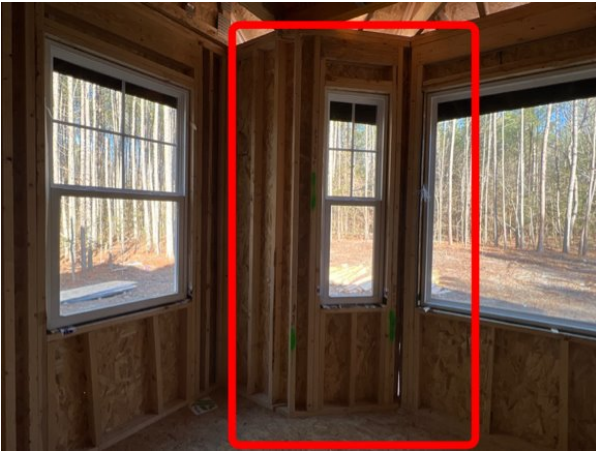
16: Missed nails noted in several areas on the exterior walls that need to be sealed.
