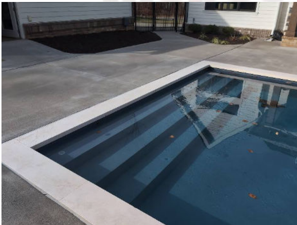
Missing handrail
