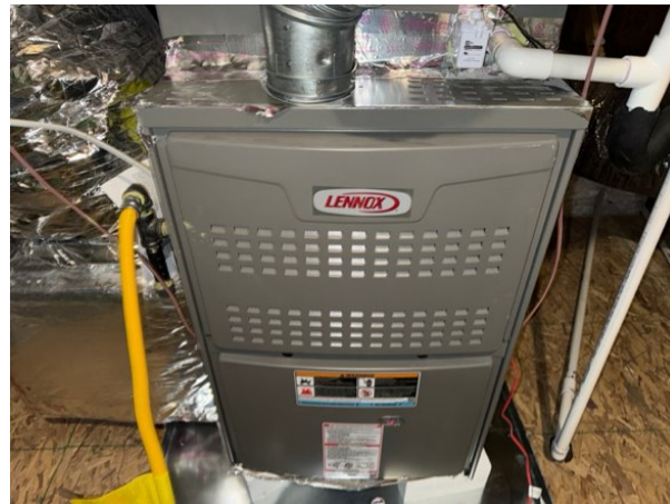
1st floor gas furnace
