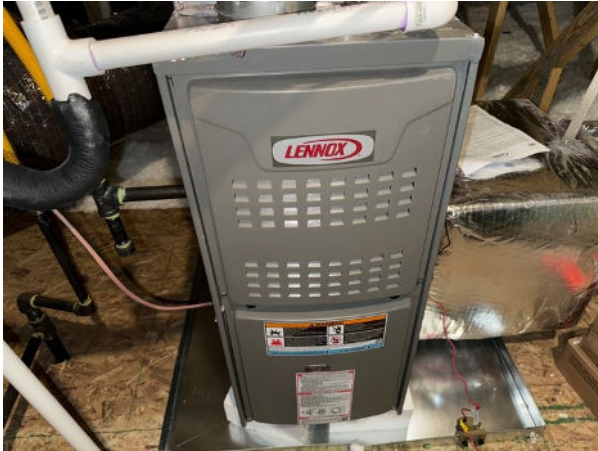
2nd floor gas furnace
