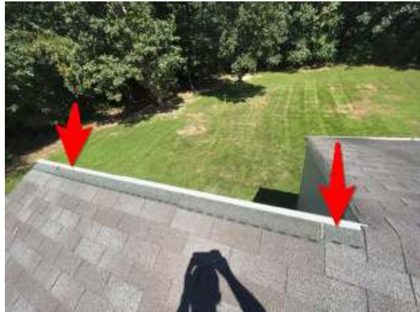
9: The roof over the addition where the ridge and rear wall meet is installed/flashed improperly. There are areas that are allowing water intrusion to occur.
