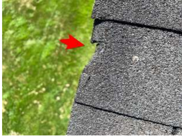
8: Cracked/damaged shingles at the right gable end of the roof.
