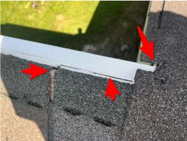
9: The roof over the addition where the ridge and rear wall meet is installed/flashed improperly. There are areas that are allowing water intrusion to occur.
