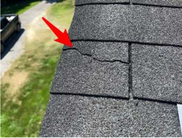
8: Cracked/damaged shingles at the right gable end of the roof.
