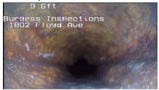
Cast Iron is rusted and corroded.
