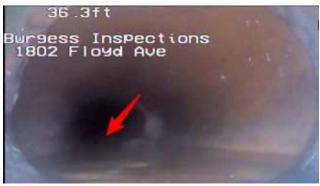
Picture show the blockage at the pipe transitions to clay.
