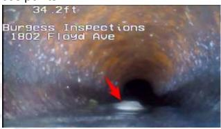
Debris in the pipe at approximately 34.5 ft from the access point
