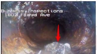
Debris in the pipe at approximately 2.4 ft from the access point
