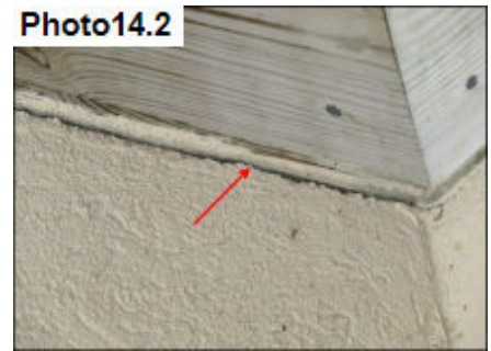
Not sealed below deck
