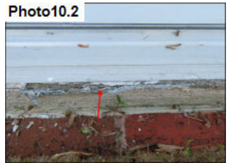
Door threshold not sealed
