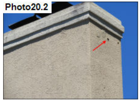
Holes need to be sealed on chimney
