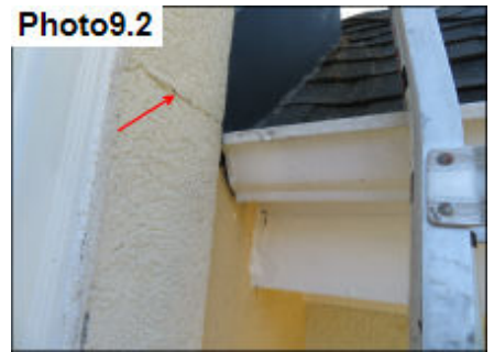
Compression crack
