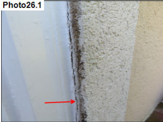
Sealant failure
