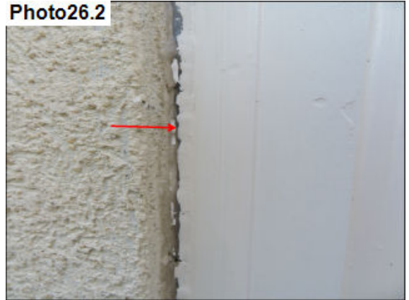
Sealant has been painted
