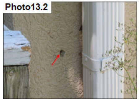
Holes from gutter downspout
